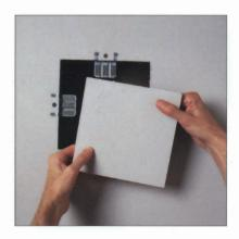
Screw through new drywall into each drywall repair clip about 3/4" from edge. Remove tabs from each drywall repair clip.
