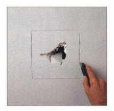
Cut a piece of drywall the size of the area of the wall to be patched. Hold that piece of drywall onto the wall and trace around it with a pencil. Carefully cut out along the pencil line and remove the damaged section of drywall.
