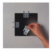
Slip drywall repair clips onto the edge of the damaged wall. Position screws about 3/4" in from edge and centre. This will line up the screws with the perforations in the clips. Screw through wall into each drywall repair clip.
