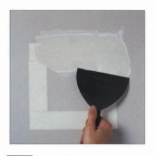
Apply CGC paper or fiberglass drywall tape and compound to patched area. Do not overlap tape. Apply second and third coats of joint compound. Allow each coat to dry before applying next, feathering out from previous coats. Sand, prime and paint when dry.
