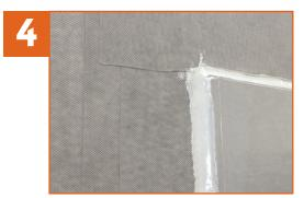
Use a compatible sealant to seal around details, reverse laps and critical areas.
